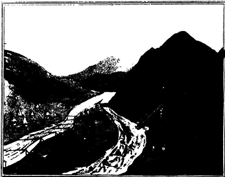
BED OF THE RIVER LAID DRY BY AN ACQUEDUCT TO COLLECT THE ALLUVIAL SOIL, IN ORDER TO WASH IT FOR DIAMONDS, GOLD, &c
