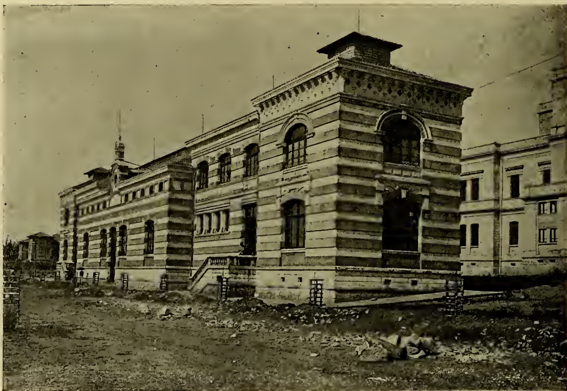
BELLO HORIZONTE — Fachada principal do Gymnasio Mineiro
